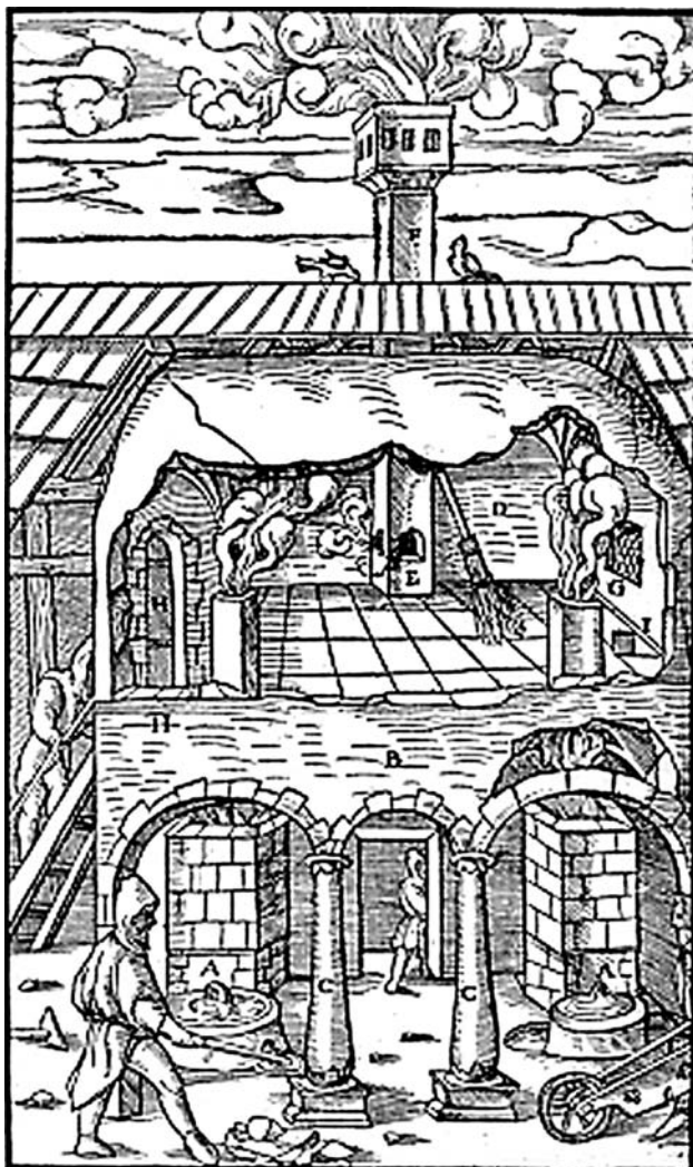
Fig. 1 Vaulted chamber built over silver smelting furnaces to collect the zinc oxide. From [24]
