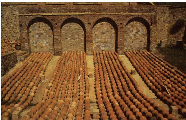
Fig. 22 View of the restored Bustamante furnace at Almadén showing the aludel condensers. From [22]
